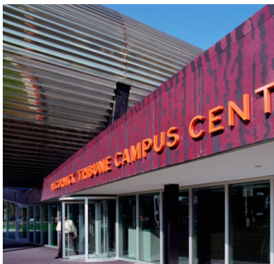
Student center signage IIT Campus Center, Chicago
