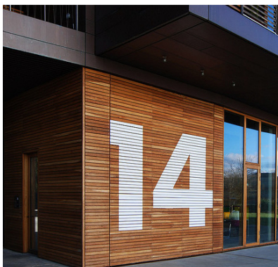
Building number, exterior Tietgenkollegiet, Copenhagen
